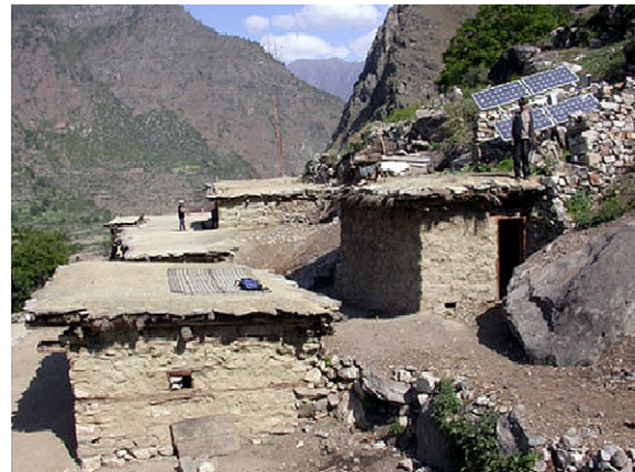
Fig. 3. RAPS Solar PV System for the remote and impoverished mountain village of Chauganphaya in Humla, Nepal [29]. A centrally built 300 W p PV array, with a two-axis self-tracking frame, developed and manufactured in Nepal, generates power for three WLED lights in 63 homes, for 6–7 h a day. All transmission cables are buried underground and able to carry a three times increased load demand over the RAPS system's cycle life of 20 years. Three local people have been trained to install, operate and maintain the system, and each household pays 15 NRp/month (~0.22 US$) for the light service (Picture: Alex Zahnd).
